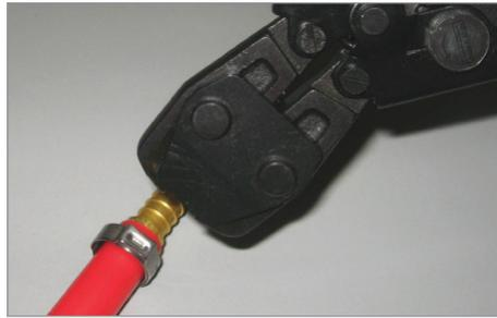
2. Slip PEX pinch clamp over tubing and insert fitting. Place pinch clamp 1/8" below edge of tubing.
